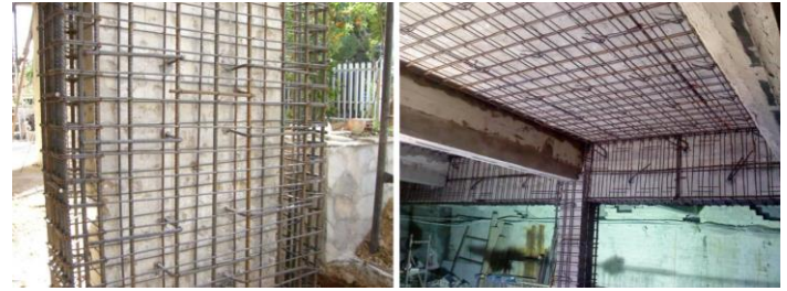
Figure 2: Diagram showing the process of applying concrete jacketing to an existing RC structural element [8] .
