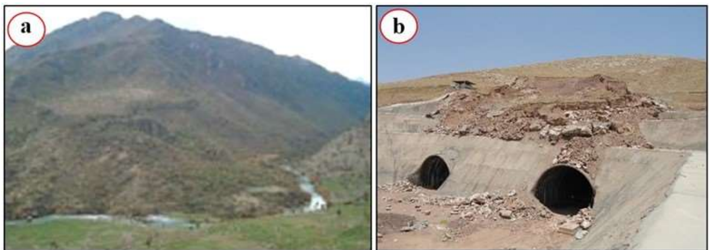
Figure 6: Landslides, a) Very old landslide along the Khabour River, note the shifted course of the river due to the landslide, b) Recent landslide (May 2015) on top of the abandoned Koya tunnel.
