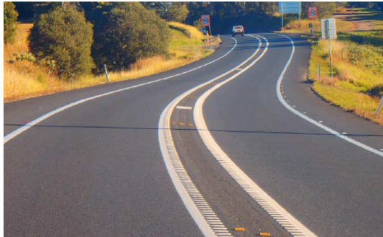
Figure 2: Continuous Painted Median Strip Installation 36
