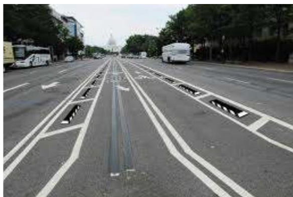
Figure 6: Rigid barrier: Cable Barriers
